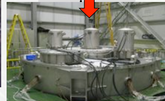
Install calibration units
